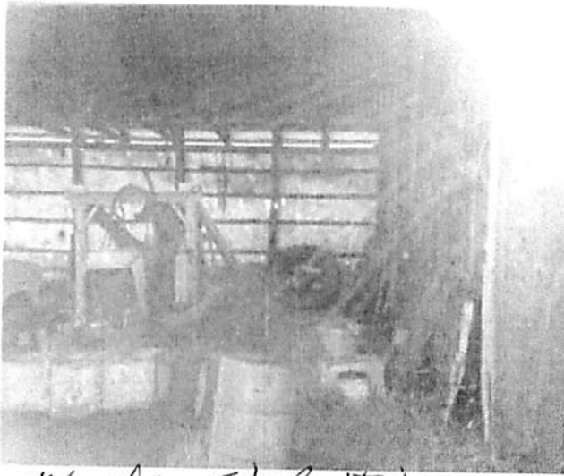
Machine Shed Tiles Iron
