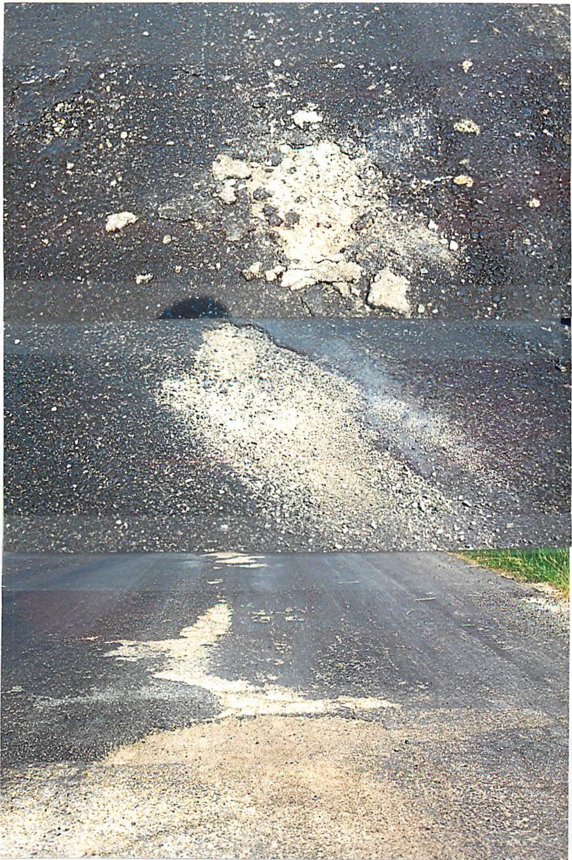
Photo #3: Taken Summer 2014 on Gold Creek Loop. This photo shows the grader asphalt patching done in the summer of 2014. Potholes were present within three weeks of patching. Did we waste our time and money?
