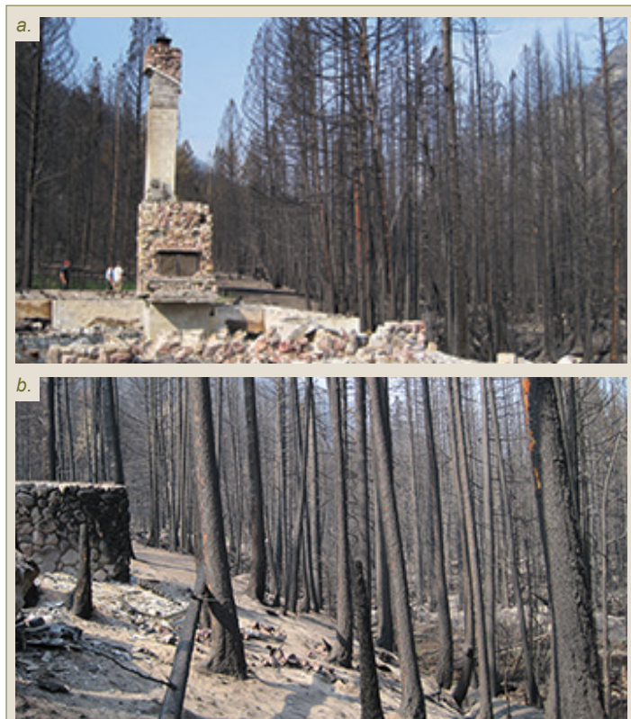
Figure 2. ACTIVE CROWN FIRE. These two separate but associated houses, a) and b) were several hundred feet apart. Both of these structures were 30 feet or closer to active crown fire.
