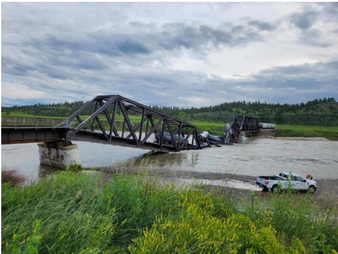
Railroad bridge collapse and train derailment on June 24 has led to closures on the Yellowstone River. FWP photo.
