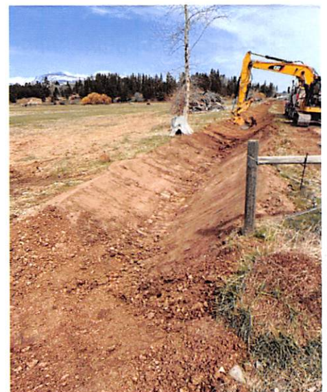
Sediment Excavation in Waddell Ditch
