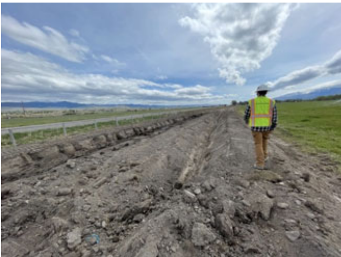
Photo from construction in summer 2021.
